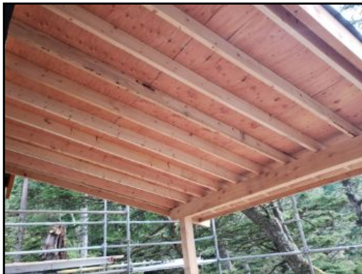
All new joists and plywood for rear roof over deck.
